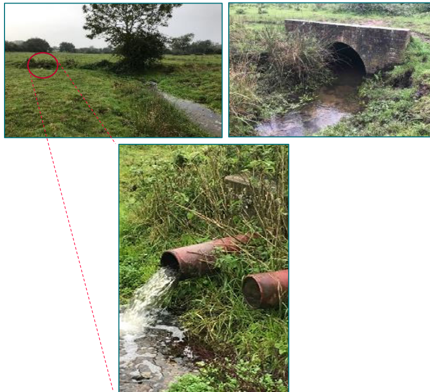
Plate 18.3.39: Outfall Pipes and Small Culvert
